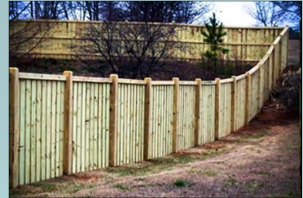
Fence with Finished Side Out
